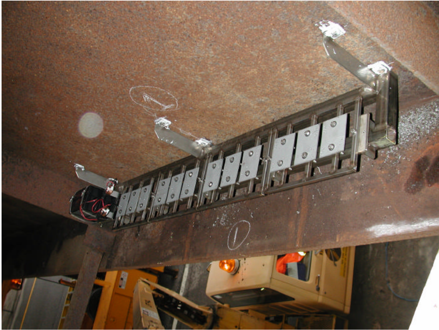
Photograph 16: Specimen Rack 1 installed (end view), at location 3CN above west abutment.
