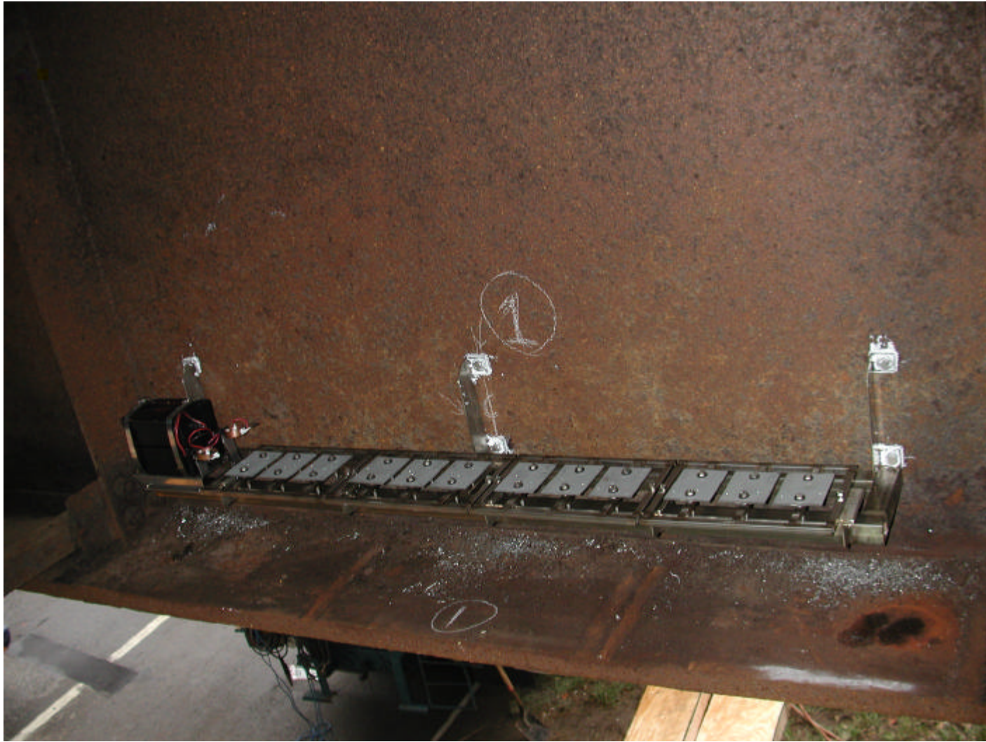
Photograph 15: Specimen Rack 1 installed. White caulking is seen at the mounting holes. Thickness measurement positions are on the flange below each end of the rack.
