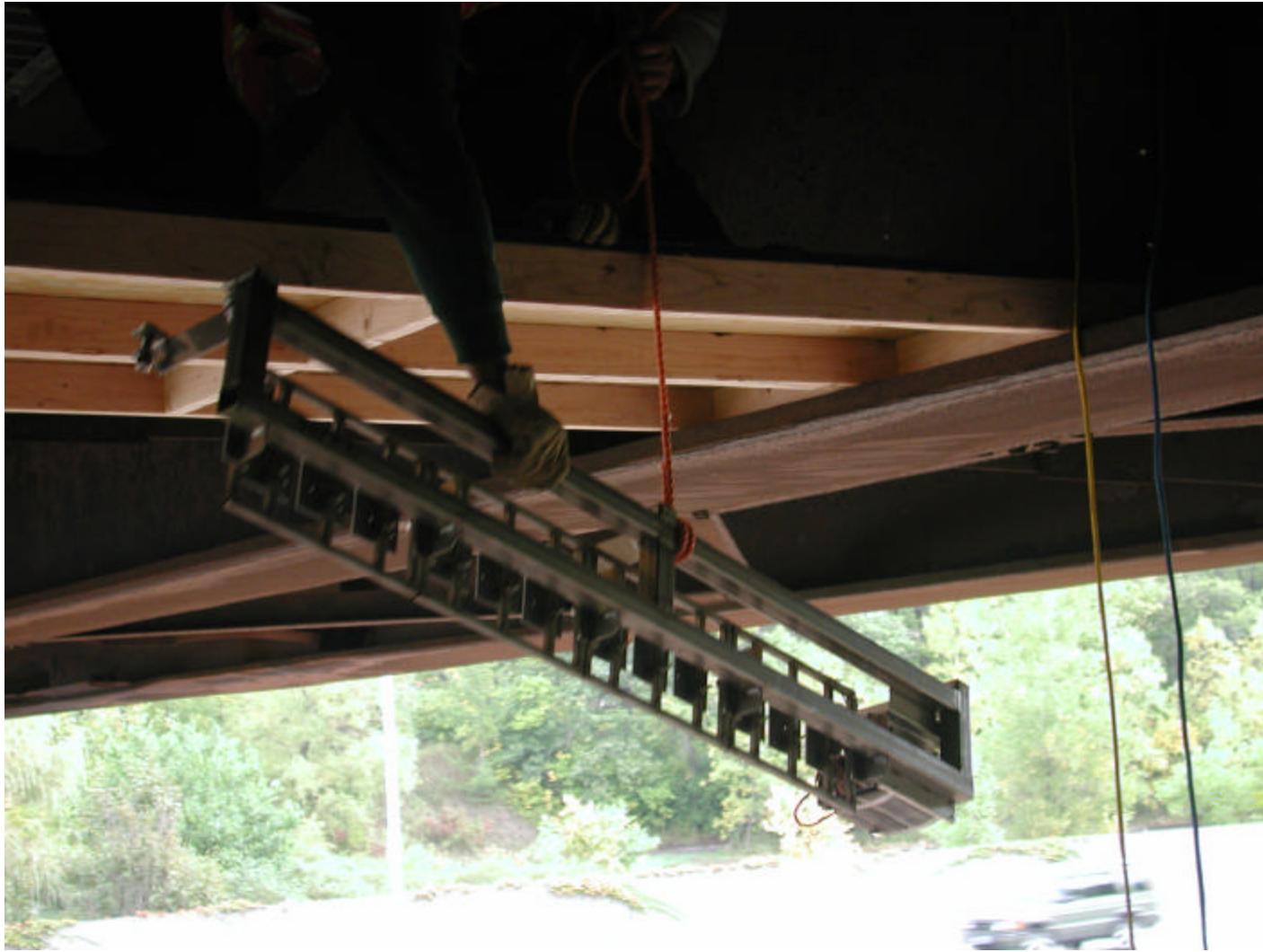
Photograph 13: Specimen Rack 2 being hoisted up to Girder 3.
